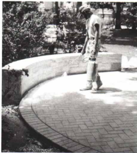
Curing compounds seal the surface of the concrete, preventing water from evaporating. In the photo above, a worker uses a garden-type sprayer to apply curing compound to a stamped concrete patio. Photo courtesy of Concrete Construction magazine.
